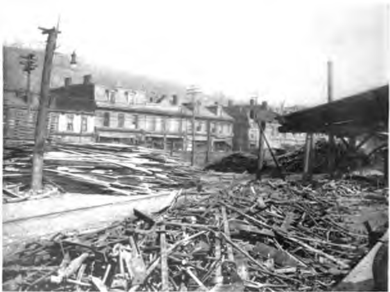
AS THE MILL SEES THE TOWN View from interior of mill yard, upon main street
